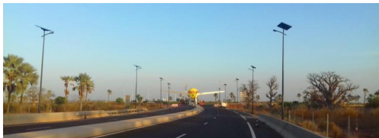
Access road at Blaise Diagne International Airport, Dakar – Fonroche Lighting.
