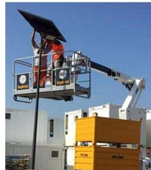
**2 Erect the mast with the assembly**
